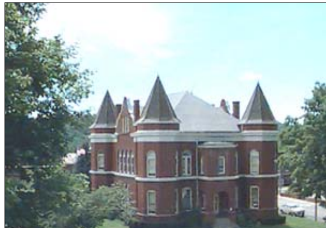
Figure VII-5. Historic 1908 Courthouse in Independence.
